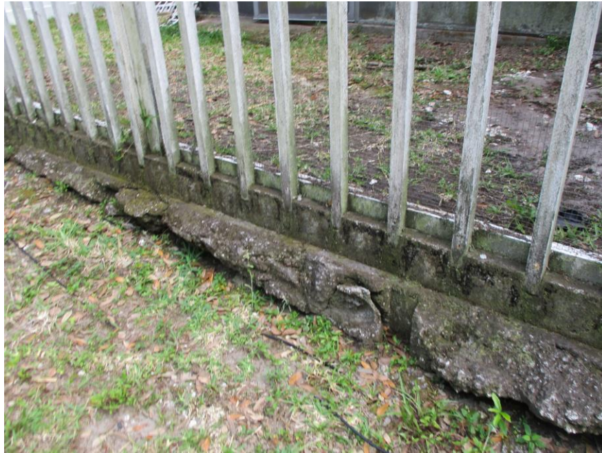
Existing Fencing supported by Concrete Footing
