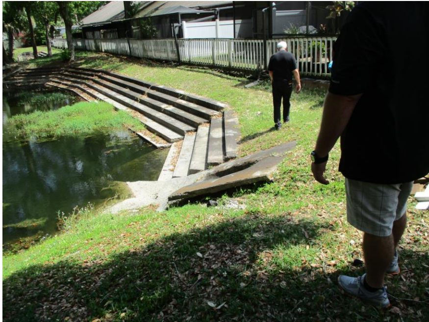
Overview of Sewall and Fence at North Elevation of Building
